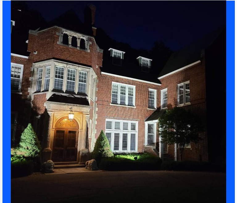
▲ Holmdene Manor is located in the center of the Aquinas College campus.
